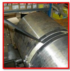
2.12 Clean for oil and dirt before applying Silicon and tape (metal cleaner, see datasheet)
