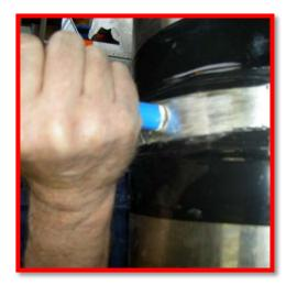
2.21 Grounding plate must be welded as close as possible, in order for the wires to be as short as possible.
