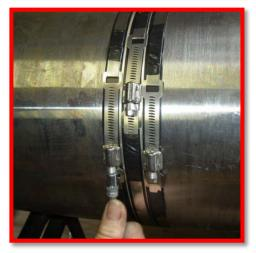
2.11 Remove the middle stainless steel band and remove el-tape
