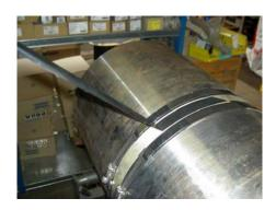
Apply silicone longitudinal on the edge of the silver band in both sides
