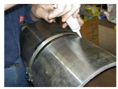
Seal the silicone with a wet finger all the way around in both sides
